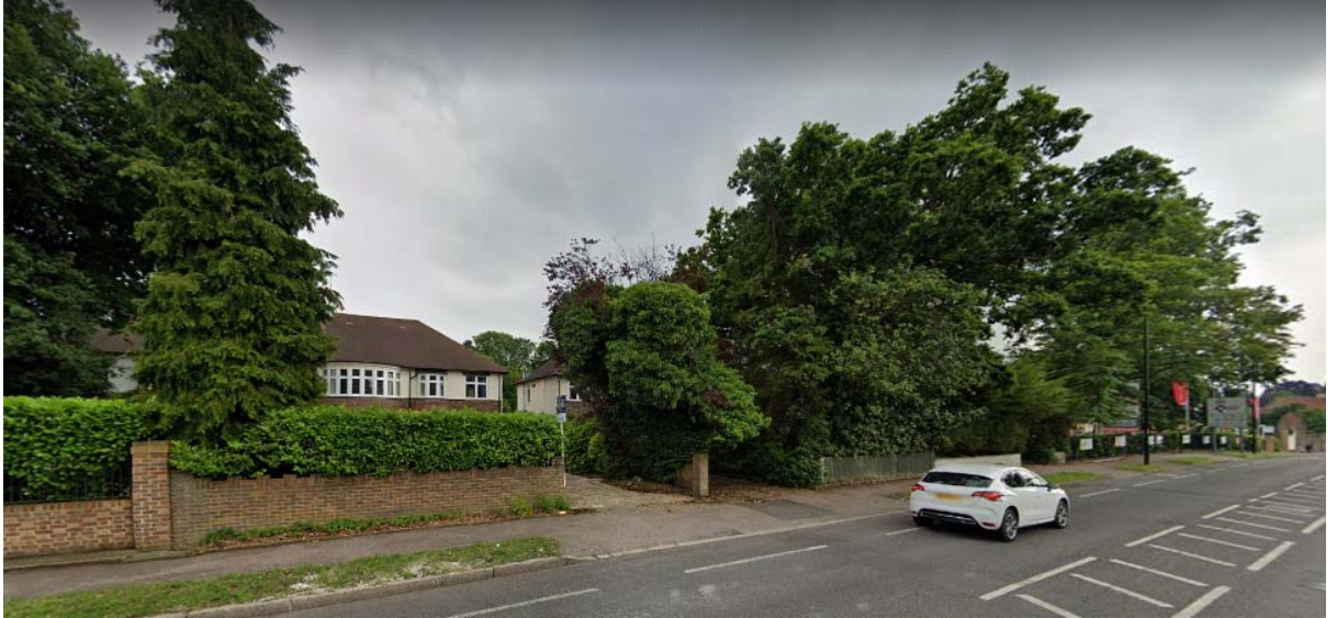
Figure 3. Frontage of 6 (adjacent site), 4 & 2 Addington Road (application site)
